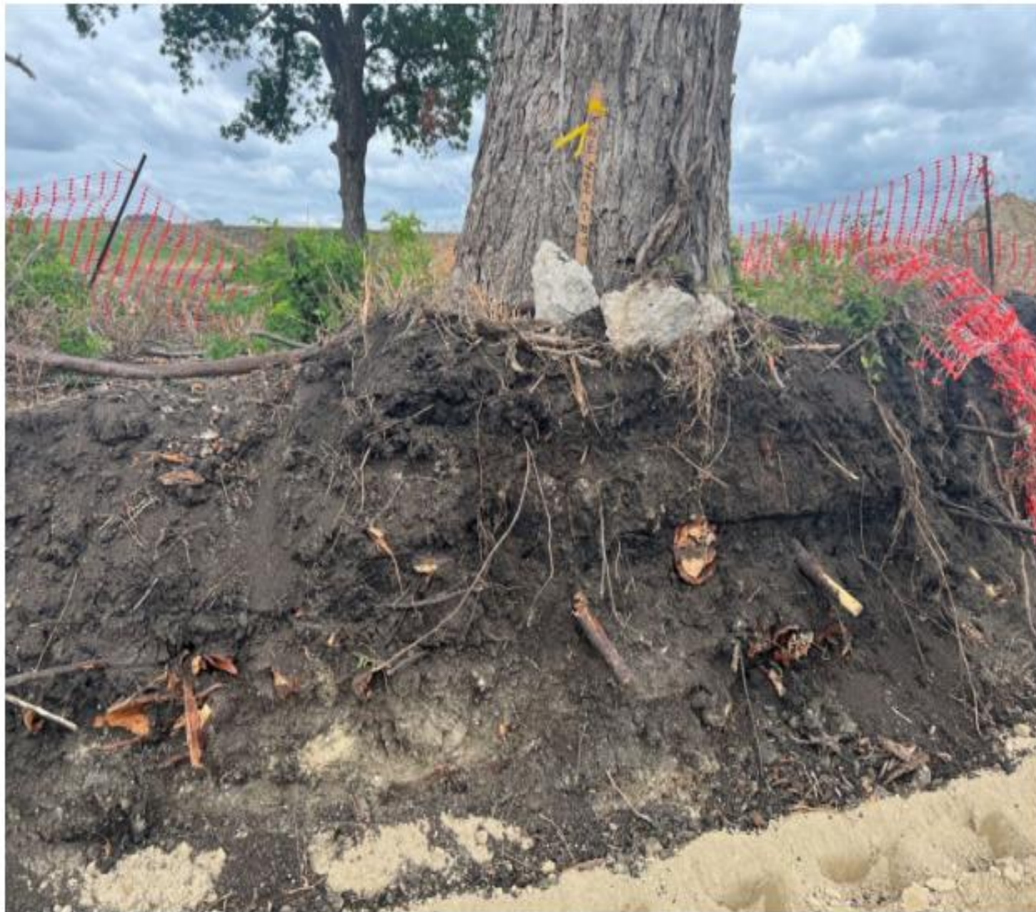
Tree 144 – significant root damage from road grade cut. Tree 146 (another pecan tree) in background demonstrates dense foliage in canopy by comparison.
