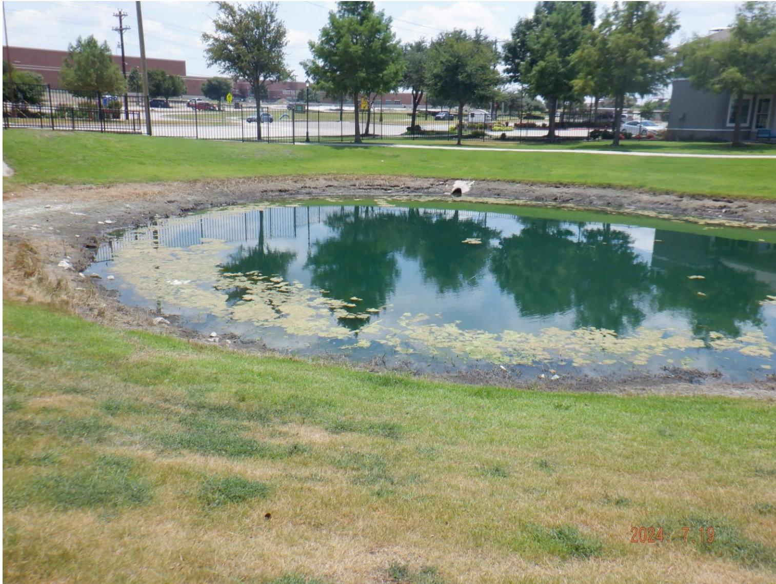
Excessive algae in a post construction feature throws off the dissolved oxygen levels of the water.
