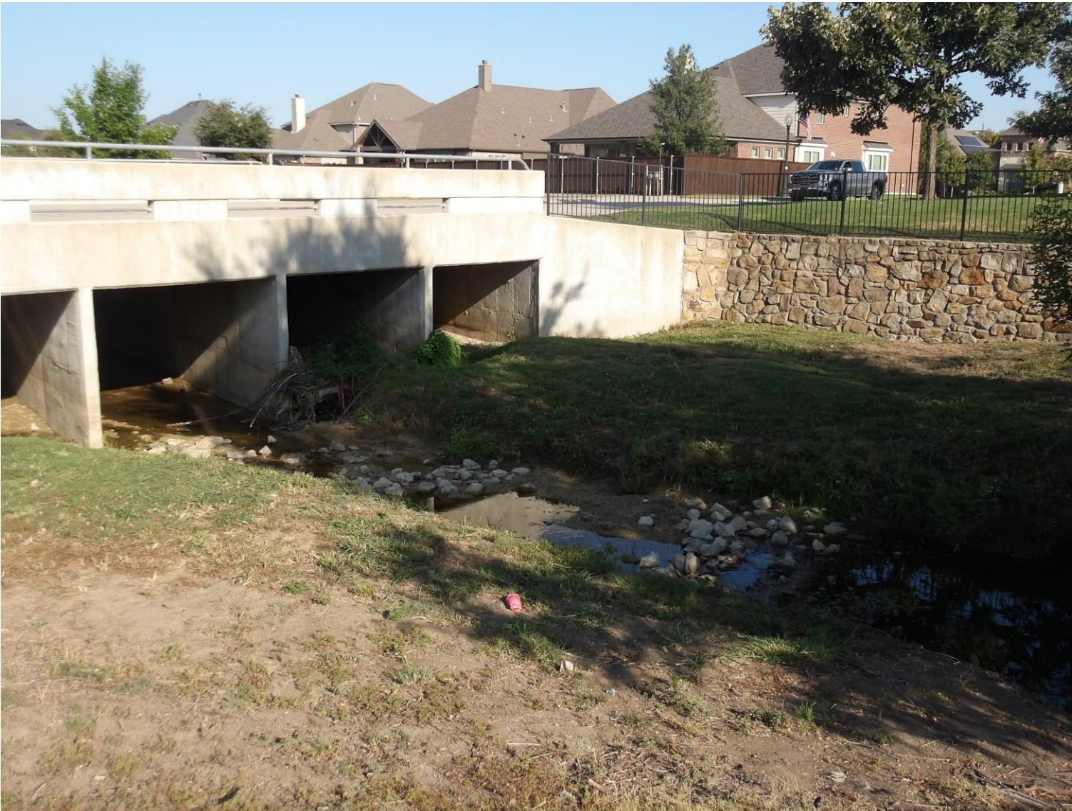
Excess sediment has blocked culverts, blocking the flow of water, which creates a flood hazard for residents and negatively impacts stream health.
