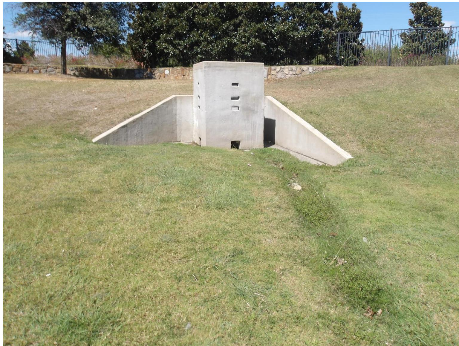
Excess sediment and vegetation that block designed drainage flumes, reduce the capacity for water, which creates a flood hazard for residents. Areas like this, also provide spots for water to pond, creating a mosquito hazard.
