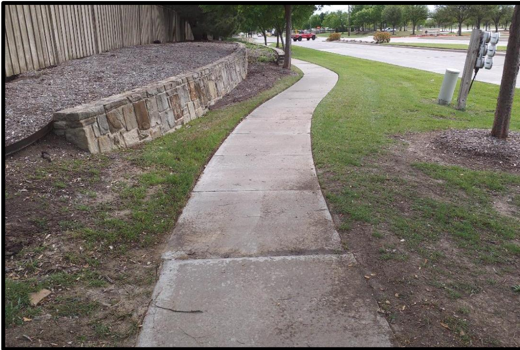
SINKING AND PONDING PROSPER TRAIL
