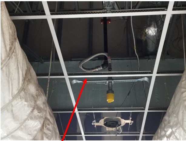
Failing to maintain the 4” minimum radius & number of bends allowed for 2’ hose in violation of the U. L. Listing
