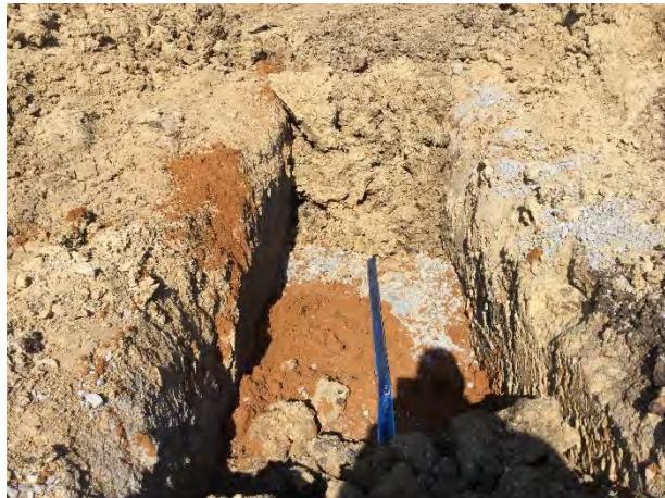
Performing the inspections of underground fire service & remote FDC installations has become progressively more difficult over the years. Safety concerns are expressed that piping may become dislodged during the hydrostatic pressure test, so contractors are backfilling natural soil to a degree the critical features for visual inspections of the piping installation are completely obstructed and cannot be verified for compliance.
