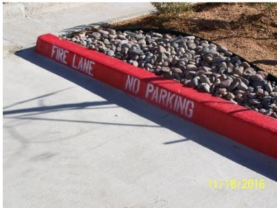
1. Striping - Fire apparatus access roads shall be continuously marked by painted lines of red traffic paint six inches (6") in width to show the boundaries of the lane. The words "NO PARKING FIRE LANE" or "FIRE LANE NO PARKING" shall appear in four-inch (4") white letters at 25 foot (25') intervals on the red border markings along both sides of the fire lanes. Where a curb is available, the striping shall be on both the horizontal and vertical faces of the curb.
